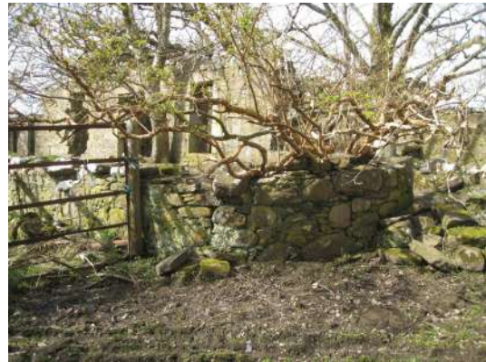
Curved wall N. End of farmhouse And gate.
