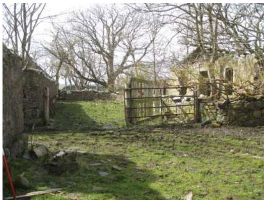
Way in and beyond, area between stables and farmhouse.
