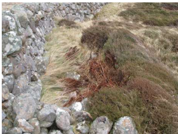
66. NG 85448 87166 elev 12m Small pen on shore side of the farm boundary wall
