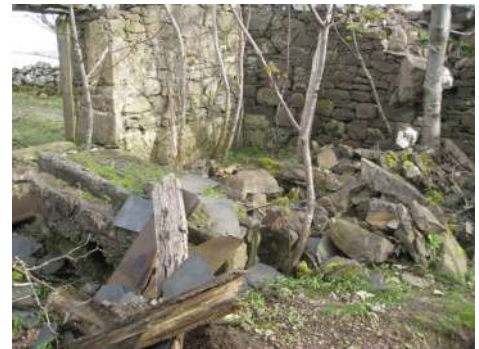
Collapsed chimney
