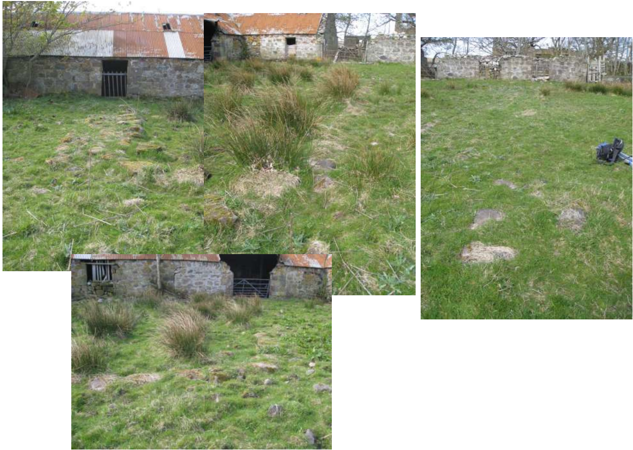
Footings within 'The Square'
