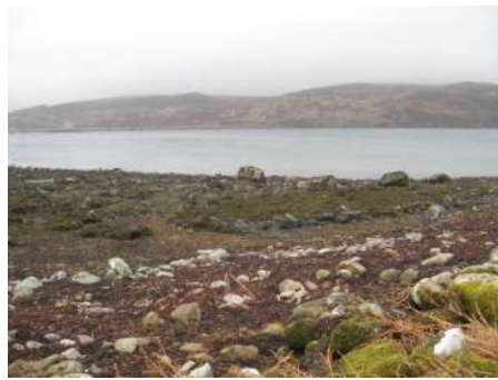
72. NG 86157 87169 elev 2m Wall and slipway on shore
