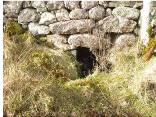
the culvert under enclosure wall at bottom end of enclosure
