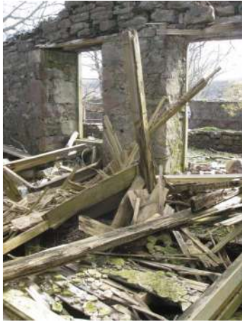
These photos show the internal side of doors and windows with collapsed timbers and plasterwork.
