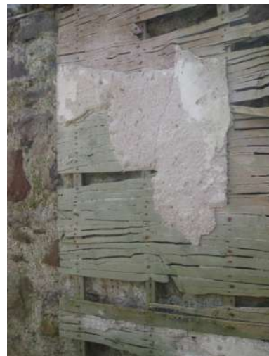
Remains of the lath and plaster walls
