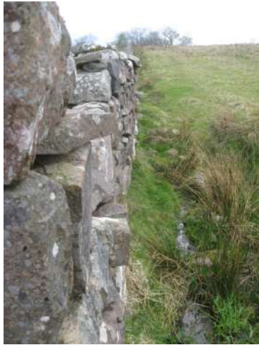
Wall lining up with enclosure wall
