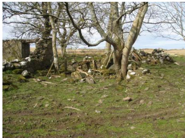
Ruinous building beside the Farmhouse.
