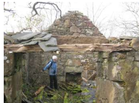
Wooden beam and slates
