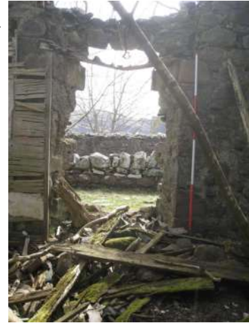
These photos show the internal side of doors and windows with collapsed timbers and plasterwork.
