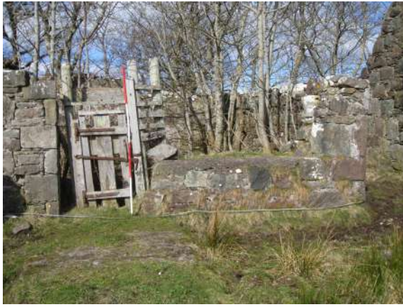
Concrete platform used for loading cattle
