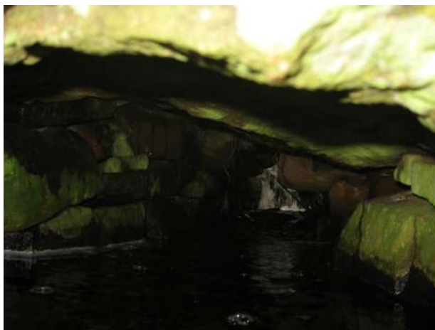
looking into the culvert at remaining stonework.
