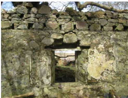
This window on the rear wall looks as if it could possibly have been altered. Was it originally an archway?
